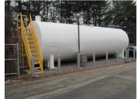
20,000 gallon oil tank located at NHS
